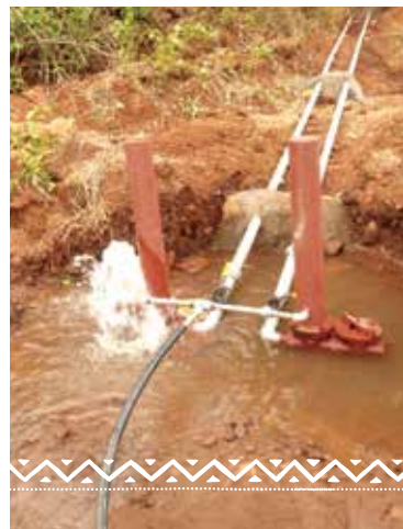
Hydrum Unit: Muvvalavariveedhi village
